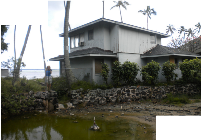
A view of the makai (ocean facing) building on the property, formerly the Lee residence at 5841 Kalaniana'ole Highway.
