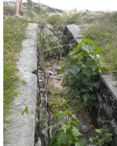
The channel and mā kāhā (sluice gate) where fish would enter the pond and spring water was expelled to the bay.
