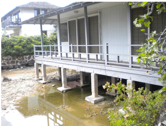
The structural piers supporting the residence.
