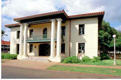
The old Lāhainā Courthouse is being renovated into a visitor orientation facility while restoring its architectural features and interpreting its history. (Source: ONMS)
