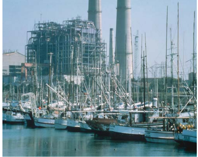
Figure HDD-1 – Moss Landing Harbor
