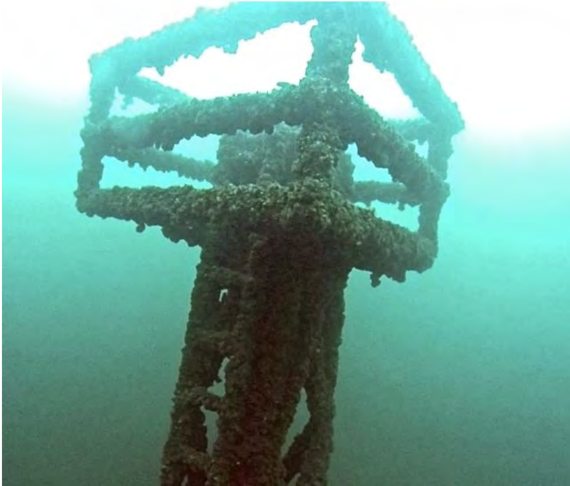
Figure 4.35. Invasive mussels covering a submerged light beacon. Photo: Tim Caza
