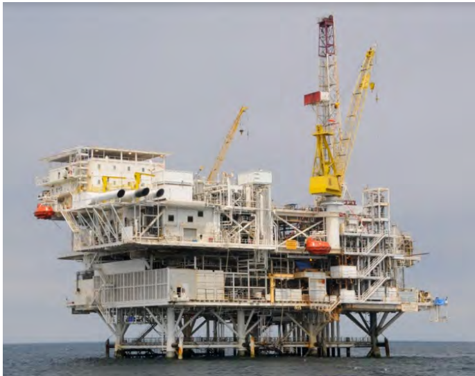
Figure R.P.2. Platform Gail, located directly adjacent to the sanctuary's north-eastern boundary area, operates at a water depth of 739 feet. Photo: R. Schwemmer/NOAA
