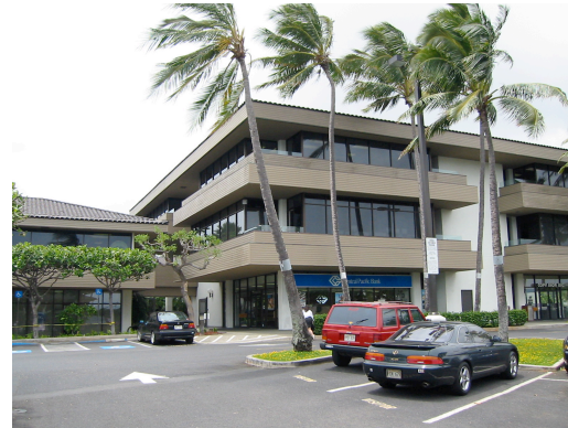
Commercial Office Building Containing new HIHWNMS and NWHICRER offices Honolulu, HI
