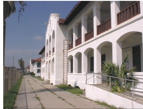
Building 302 NMFS Galveston Laboratory Galveston, TX
