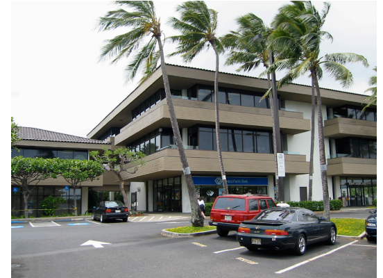
Exterior of office building now housing NWHICRER. Space to be shared with HIHWNMS staff offices. Honolulu, HI
