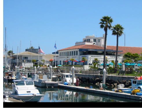
Santa Barbara Marina. Large Tile Roof Building is Maritime Museum . CINMS Headquarters is located on rear side of Museum
