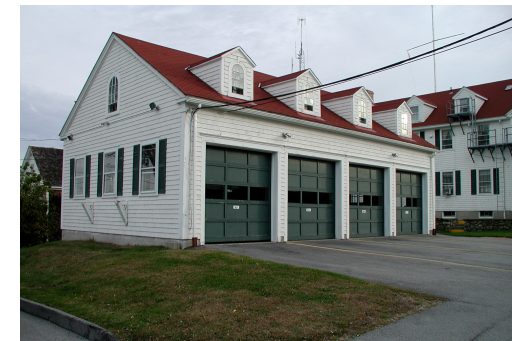
SBNMS garage at rear of headquarters building, proposed as meeting facility, Scituate, MA
