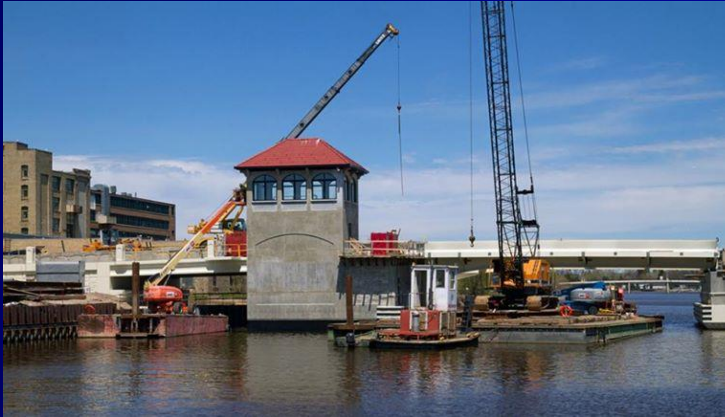
Replacement of the 17th Street lift bridge, 2012-13
